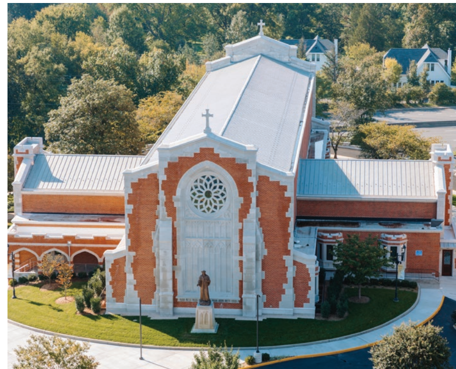
Renovation of Saint Thomas More Cathedral (Arlington)
